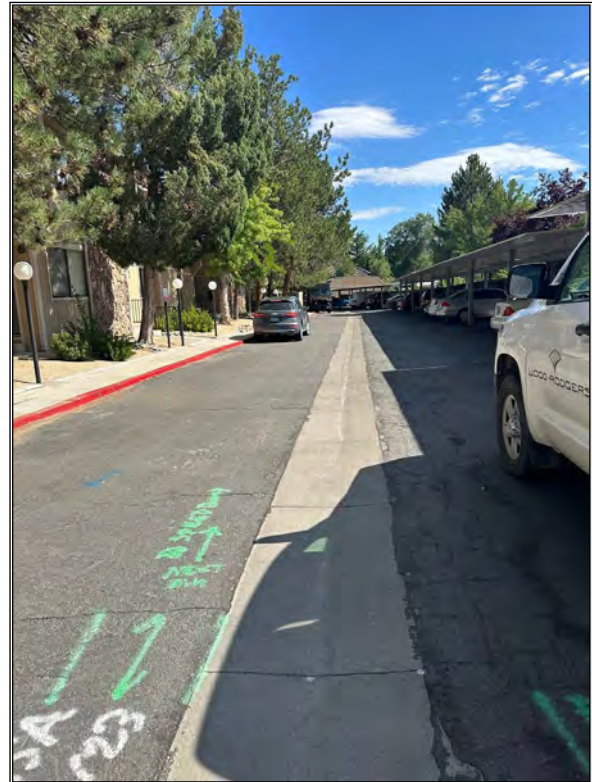
IMAGE 2: Valley Gutter along East Side of Site
