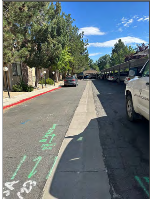
IMAGE 2: Valley Gutter along East Side of Site
